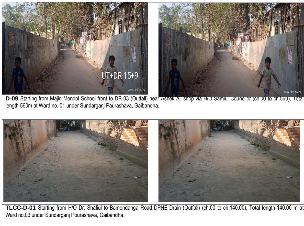
Figure 3:Existing Roads and Drains Picture
